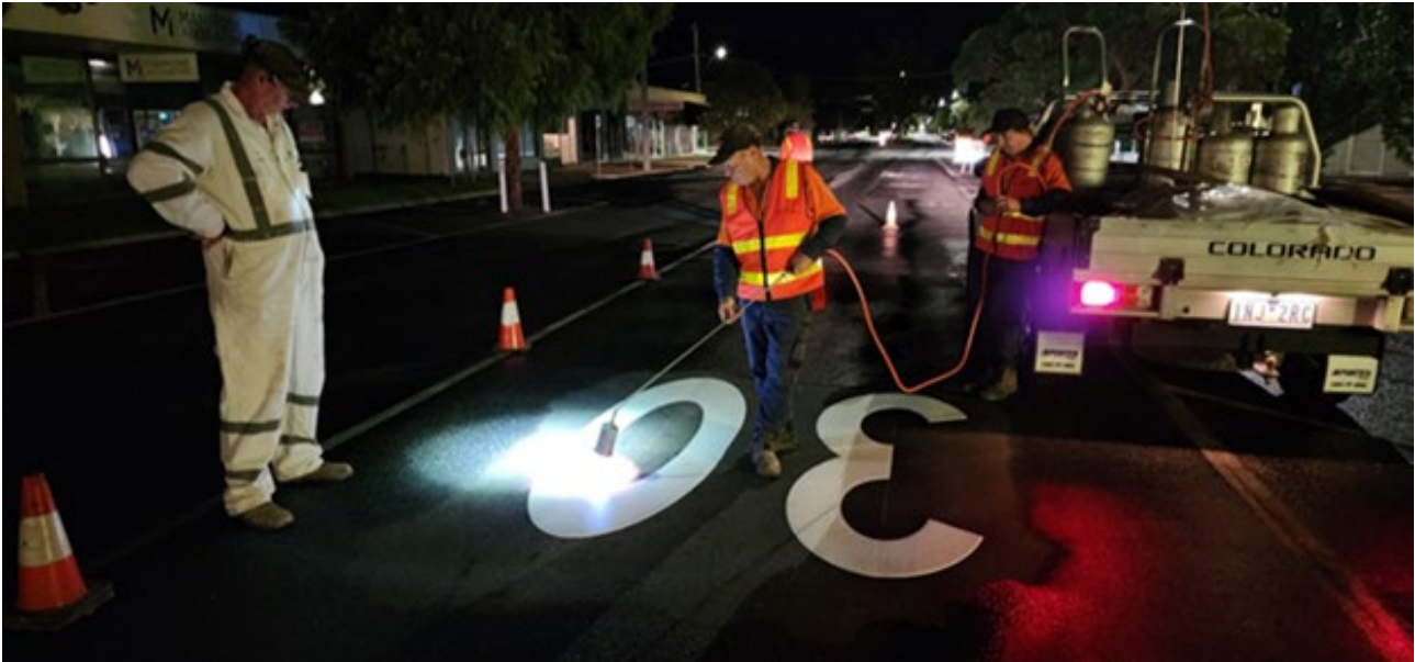
Figure 2.9: Installation of Thermoplastic pavement markings in Mildura
